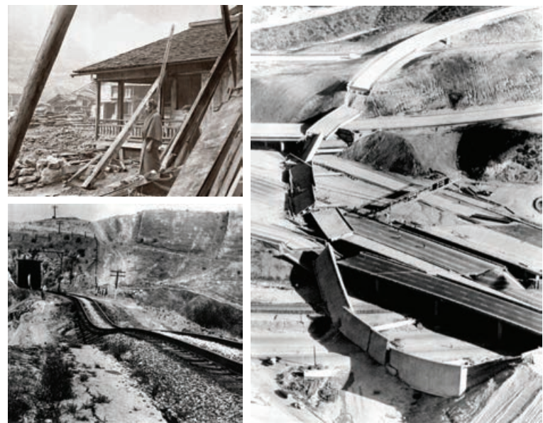
Damage caused by earthquakes
