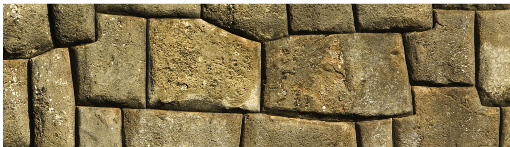
Tightly wedged stones
