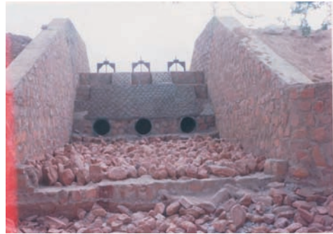
Turra dam: view for upstream side
